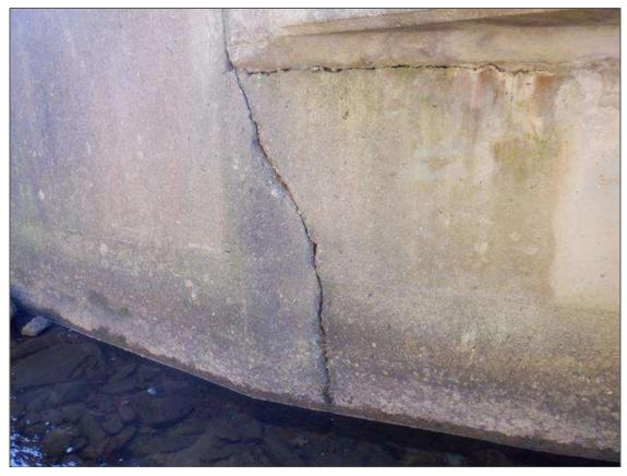
Barrel 4 - RCBC Barrel 4: FULL HEIGHT X 0.5 INCH WIDE VERTICAL CRACK IN EXTERIOR WALL AT UPSTREAM END OF THE BARREL.
