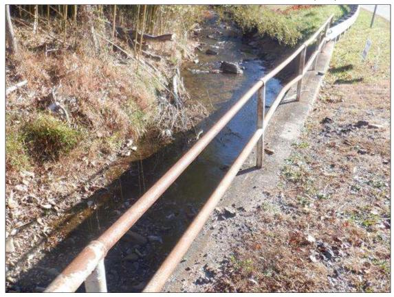
Span 2 - Slab Steel Rail 1: TWO POSTS LEANING WESTWARD 1 INCH AT THE TOP, AND BOTH RAILS ARE BENT AT FAR END OF THE SPAN.
