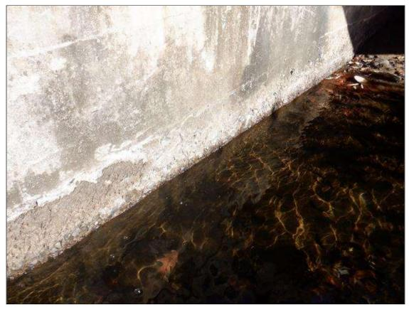
Pier 1 Pier Wall: ABRASION 1 FOOT HIGH X 20 FEET LONG BEGINNING AT THE RIGHT END WITH COARSE AGGREGATE INTACT.
