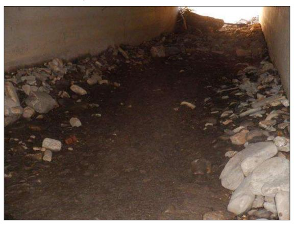
ROCK AND SEDIMENT BUILDUP UP TO 2 FEET DEEP IN ALL BARRELS.
