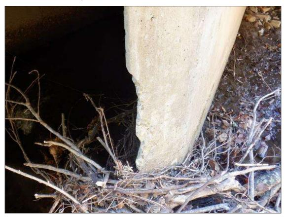
Barrel 4 - RCBC Barrel 4: SPALLS IN THE UPSTREAM END OF INTERIOR WALL 3 UP TO 1 INCH DEEP.
