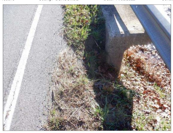
EROSION CAUSED BY STORMWATER RUNOFF AT THE SOUTH EAST CORNER 3 FEET WIDE X 6 FEET LONG X 1 FOOT DEEP CURRENTLY AT THE EDGE OF PAVEMENT. (PAR)
