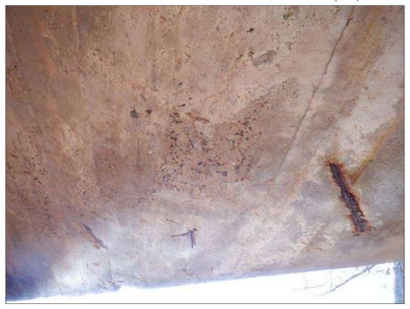
Span 1 - Slab Slab 1: NUMEROUS SPALLS ALONG RIGHT SIDE UP TO 6 INCHES IN DIAMETER WITH EXPOSED AND CORRODING REBAR WITH MEASUREABLE SECTION LOSS. (PAR)
