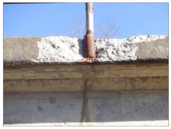
Span 1 - Slab Right Rail: 3 FEET WIDE X 9 INCH HIGH X 3 INCH DEEP SPALL OF THE CONCRETE AT THE BASE OF POST 5. THE ANCHOR OF THE POST IS COMPLETELY EXPOSED AND LOOSE. (PAR)
