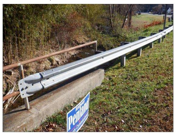
APPROACH RAILING AT NORTH WEST AND SOUTH EAST CORNER IS CONNECTED TO BRIDGE RAIL BY ONE U BOLT.
