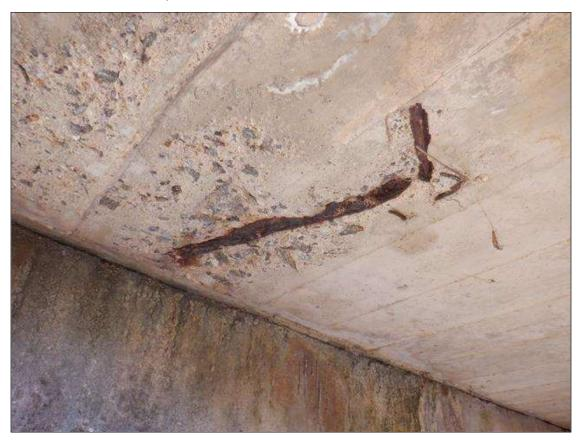
Span 2 - Slab Slab: SPALL IN BOTTOM FACE 2 FEET LONG X 9 INCHES WIDE X 1 INCH DEEP WITH REINFORCING STEEL EXPOSED WITH MEASUREABLE SECTION LOSS AT NEAR END, 2 FEET FROM RIGHT EDGE. (PAR)
