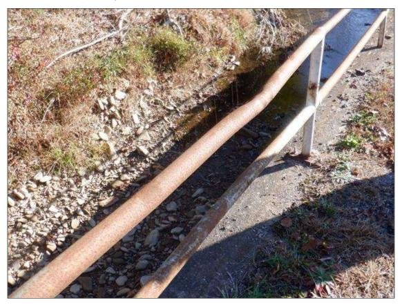
Span 2 - Slab Steel Rail 1: SURFACE CORROSION ON POSTS AND RAILS THE FULL LENGTH.
