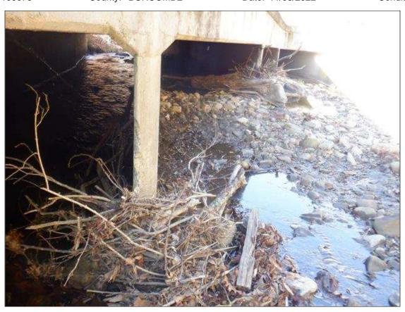
DRIFT 6 FEET WIDE X 3 FEET HIGH X 1 FOOT DEEP AGAINST EACH INTERIOR WALL.
