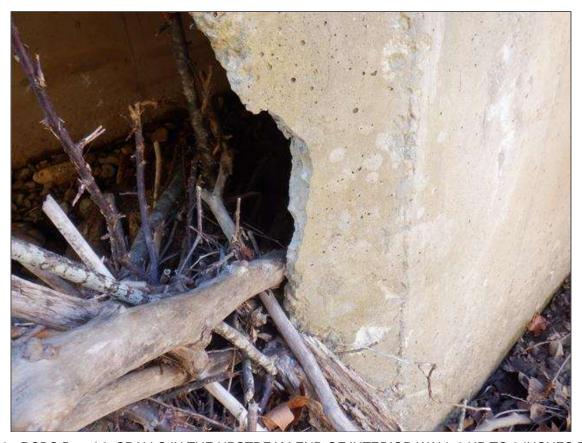
Barrel 3 - RCBC Barrel 3: SPALLS IN THE UPSTREAM END OF INTERIOR WALL 2 UP TO 3 INCHES DEEP.
