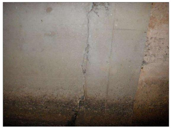
Barrel 4 - RCBC Barrel 4: FULL HEIGHT X 0.5 INCH WIDE VERTICAL CRACK IN EXTERIOR WALL AT DOWNSTREAM END OF THE BARREL.
