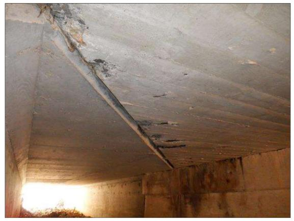
Span 1 - Slab Slab 1: NUMEROUS SPALLS UP TO 1 FOOT DIAMETER X 0.5 INCHES DEEP ALONG THE LEFT SIDE, SOME WITH EXPOSED REINFORCING. (PAR)
