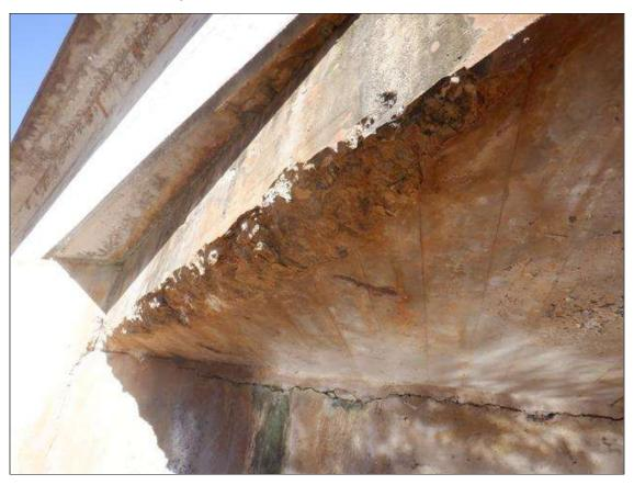
Span 1 - Slab Slab 1: 8 FEET LONG X 1 FOOT WIDE X 2 INCH DEEP SCALING DUE TO CONCRETE DETERIORATION AT THE RIGHT SIDE, NEAR END.
