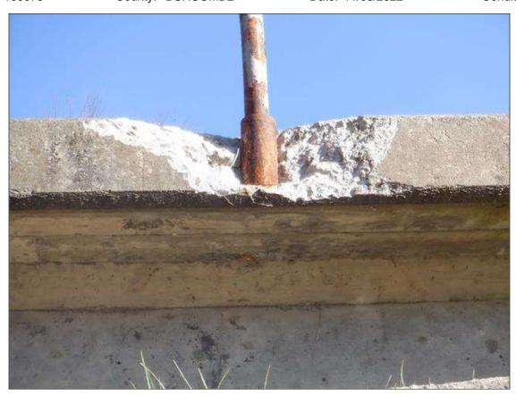
Span 1 - Slab Right Rail: 2.5 FEET WIDE X 9 INCH HIGH X 3 INCH DEEP SPALL OF THE CONCRETE AT THE BASE OF POST 6. THE ANCHOR OF THE POST IS COMPLETELY EXPOSED AND LOOSE. (PAR)
