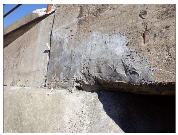
Span 2 - Slab Slab: 2 FEET LONG X 1 FOOT HIGH UNSOUND PATCH IN THE RIGHT FACE, NEAR END.
