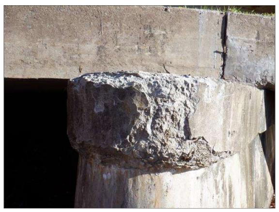
Pier 1 RC Cap: 3 FEET LONG X 1 FOOT HIGH X 2 INCH DEEP SCALING DUE TO CONCRETE DETERIORATION AT THE RIGHT END OF THE CAP.
