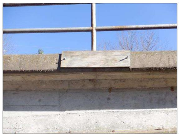
Span 1 - Slab Right Rail: PATCH TO BASE OF RAIL AT POST 4 WITH PLYWOOD FORM LEFT IN PLACE AS REPAIR TO PREVIOUS PAR.
