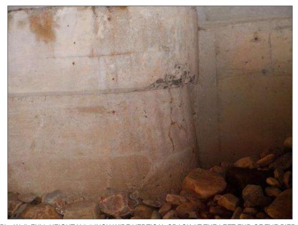
Pier 1 Pier Wall: FULL HEIGHT X 0.5 INCH WIDE VERTICAL CRACK AT THE LEFT END OF THE PIER WALL.
