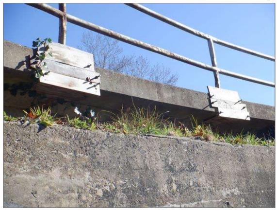
Span 2 - Slab Steel Rail 2: PATCH WITH PLYWOOD FORMS AND A STEEL PLATE AT THE BASE OF POSTS 7 AND 8 AS REPAIRS TO PREVIOUS PARS.
