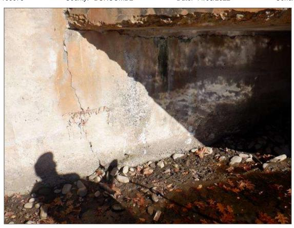
End Bent 1 Abutment: FULL HEIGHT X 0.5 INCH WIDE VERTICAL CRACK AND 13 FEET LONG X 0.5 INCH WIDE HORIZONTAL CRACK AT THE RIGHT END OF THE ABUTMENT. (PAR)
