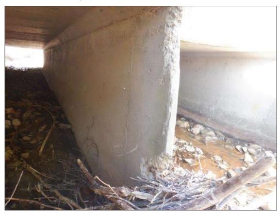
Barrel 2 - RCBC Barrel 2: SPALLS IN THE UPSTREAM END OF INTERIOR WALL 1 UP TO 3 INCHES DEEP.
